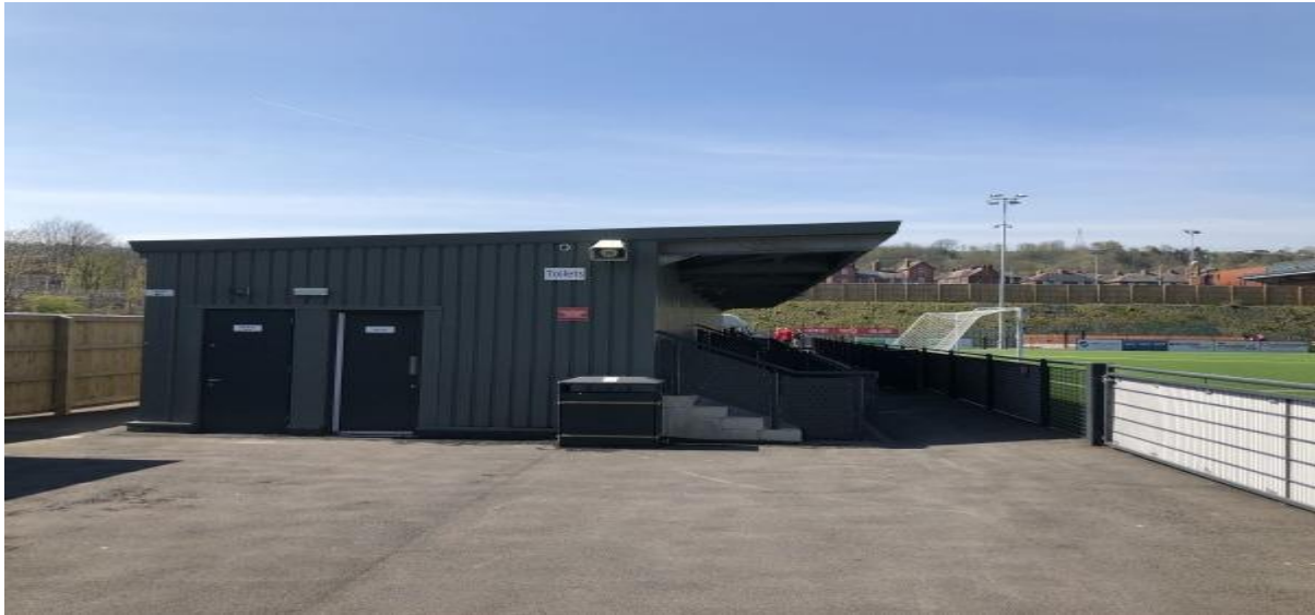
Railway Lane Enclosure
